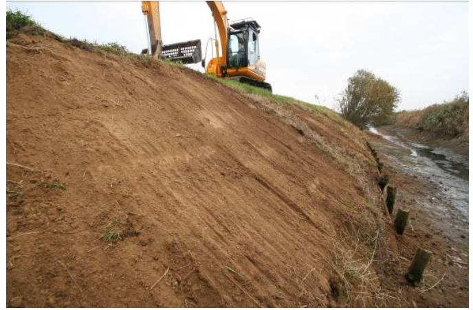
A Benwick IDB ditch with badger setts present, before and after licensed reprofiling.
