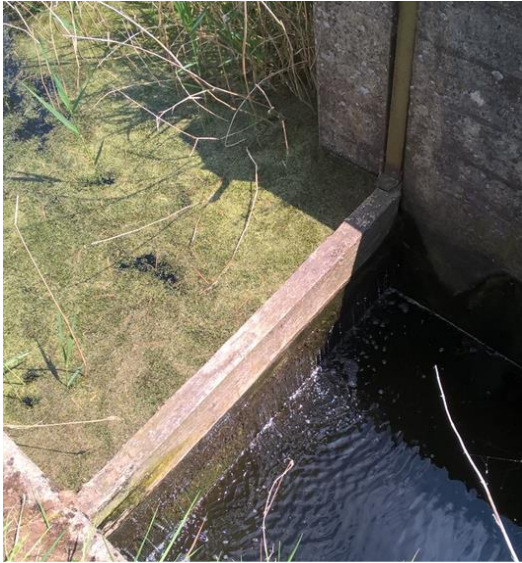
Water Control Structure Point 75
