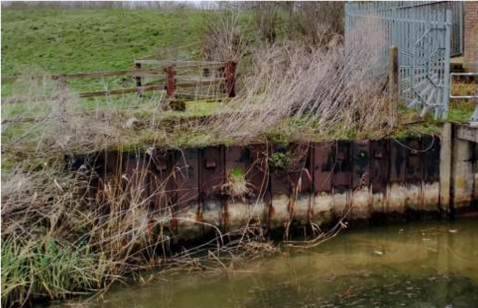
The inlet bay is constructed of reinforced concrete and appears to be in good condition. There is a 1.2 metre high galvanised post and rail hand rail around the inlet which is in good condition with a residual life of 30 years.
