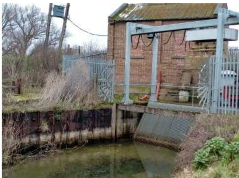
A new weedscreen and cleaner were installed in 2017 and should provide at least another 10-12 years before any major works are required.
