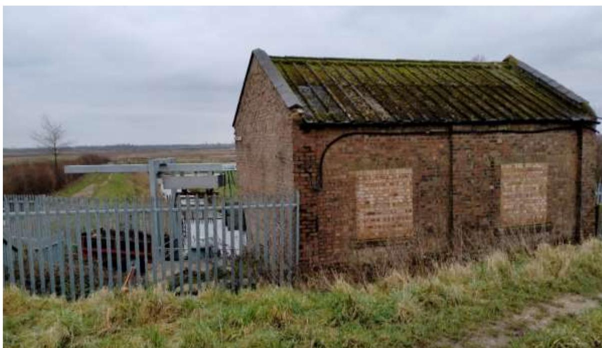
The control building is of brick construction with a corrugated roof on a steel framed trussed rafter. The roof material is likely to be asbestos and there are areas of damage which are liable to let in rain. The windows have been removed in the past and the openings have been bricked up. The building has significant frost damage and gable end ridge tiles are missing which is contributing to the problem.
