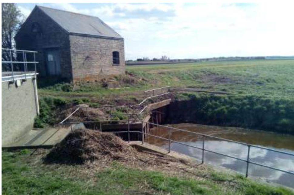
In order to maximise the life of the recently installed steel sheet piles, the Board may wish to consider coating the exposed steel with a suitable metal paint. This will serve to minimise oxidation of the steel in future years.
