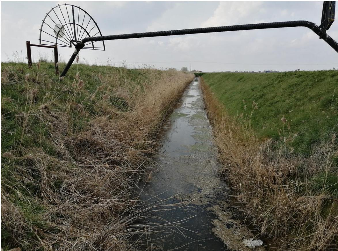
**Figure 1** Drain at node 88 showing an alternate margin cut
